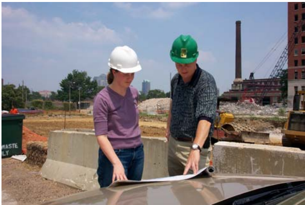
Construction Field Oversight at 10 th & Broadway
