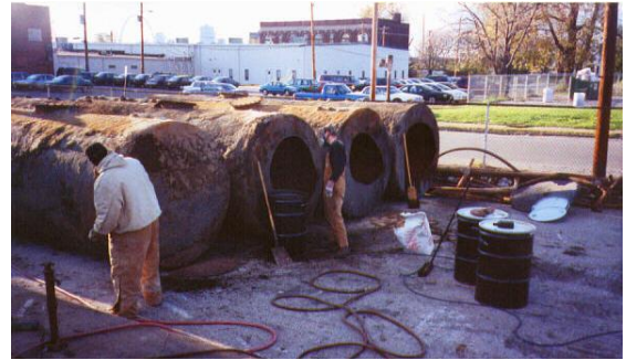
Gasoline UST Removals Conducted at 10 th & Broadway
